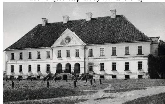
Fig. 3. Manor house Schleck.
